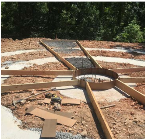
Early Construction of Rock Garden Foundation.
